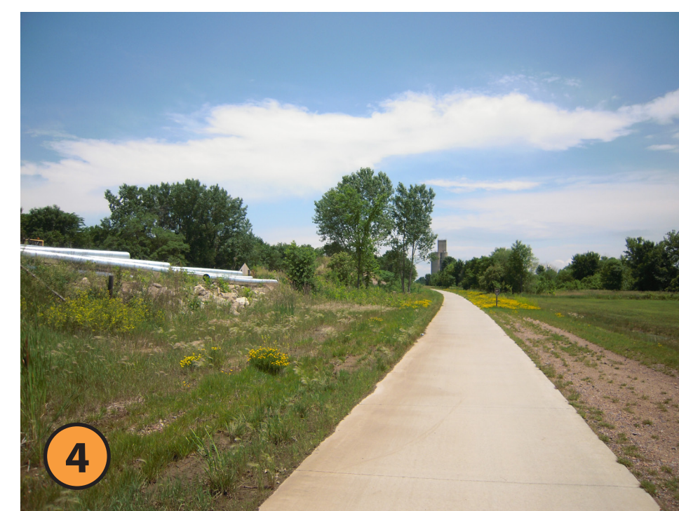
Existing Trail Corridor. Source: Nate Schlorholtz
